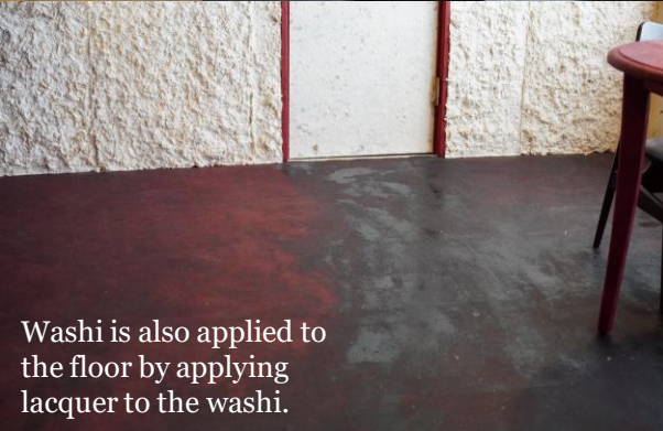
Washi can be applied to doors as well as walls.
